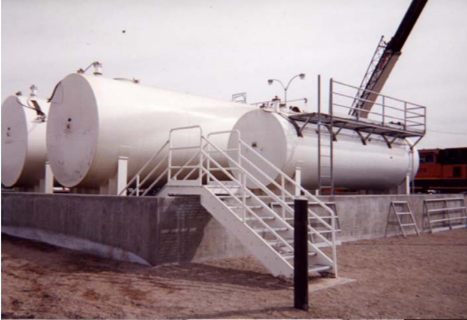
Two 30,000 gallon and one 5,000 gallon UL142 tanks on saddles.
