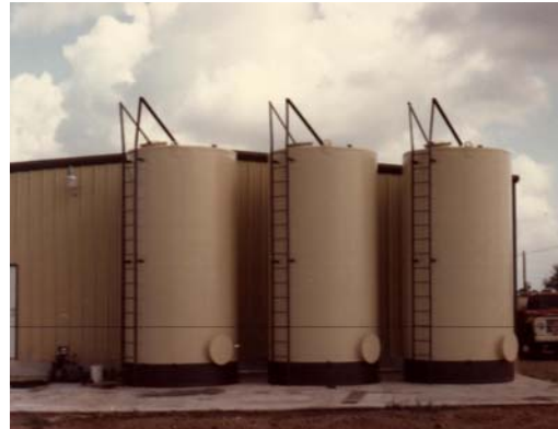
Standard API 650 tanks with ladders.
